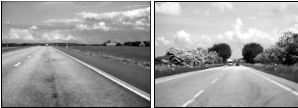
Figure 7 Roadsides can vary considerably between different landscapes and countries. Left: Road verges along a motorway in southern Sweden consisting only of an open ditch. Toxins and salt from the road surface can easily spread onto the adjacent agricultural field. Right: Densely vegetated roadsides along a highway in Germany. Bushes and trees along roads provide nesting sites to birds and screen the road and its traffic from the surrounding landscape. Fotos: A.Seiler.
